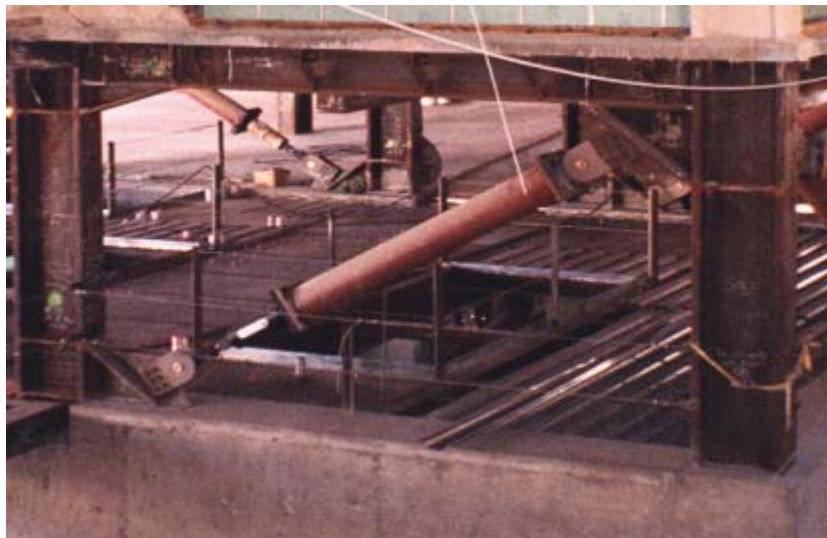
FIGURE 13: DIAGONAL BRACE FVD CONFIGURATION; PHOTO COURTESY OF TAYLOR ET AL.
